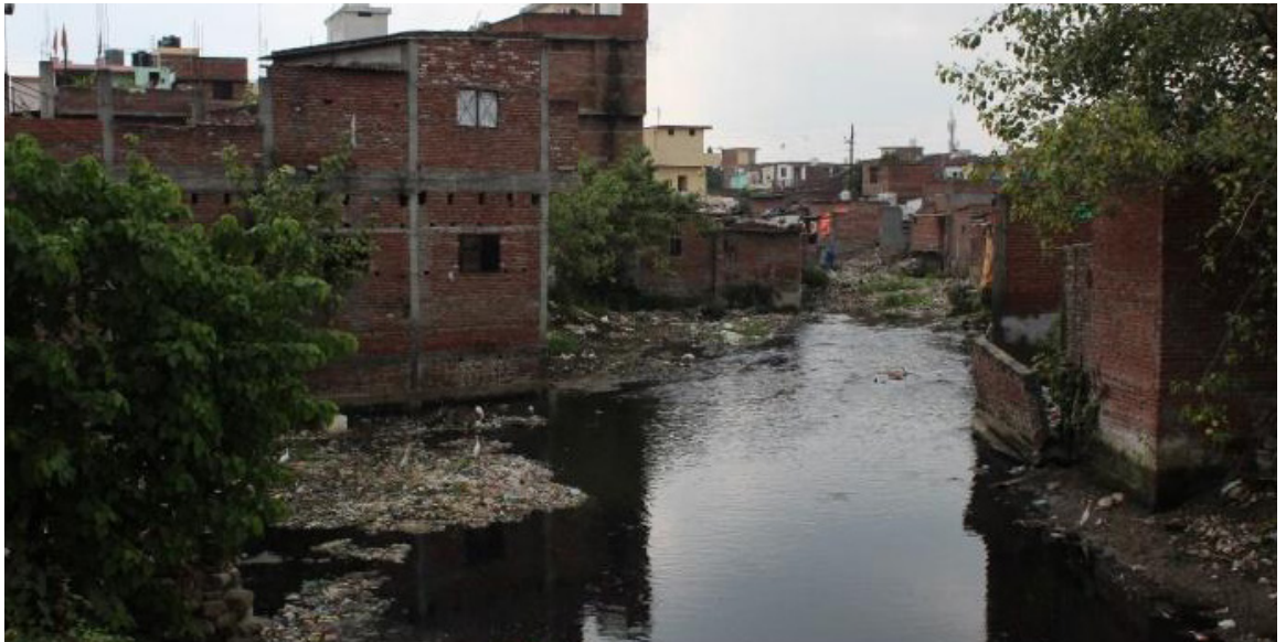
Figure 29: Kalyani river site encroachment
